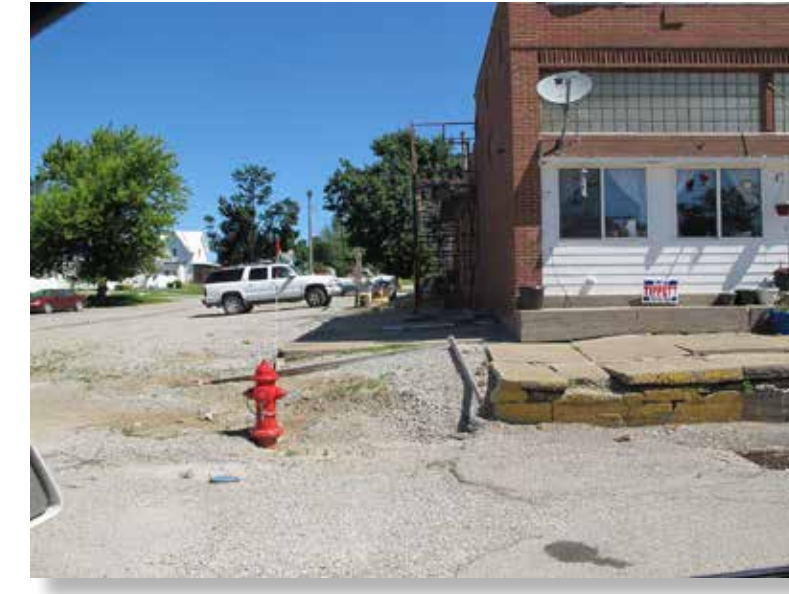
Existing conditions: Poor accessibility.
