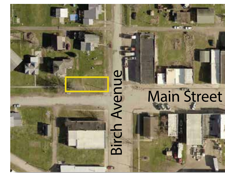
Existing aerial view.
