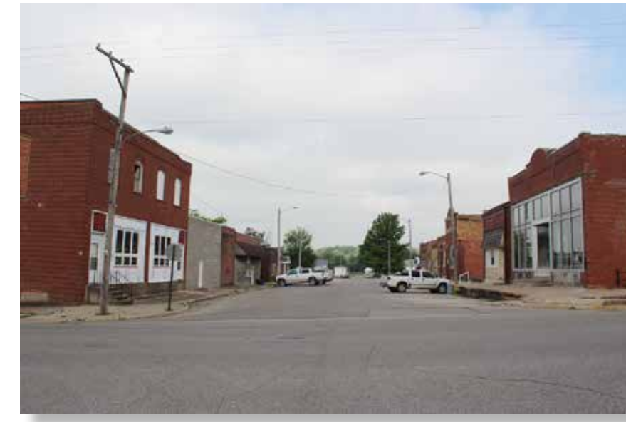
Existing conditions downtown Main Street.
