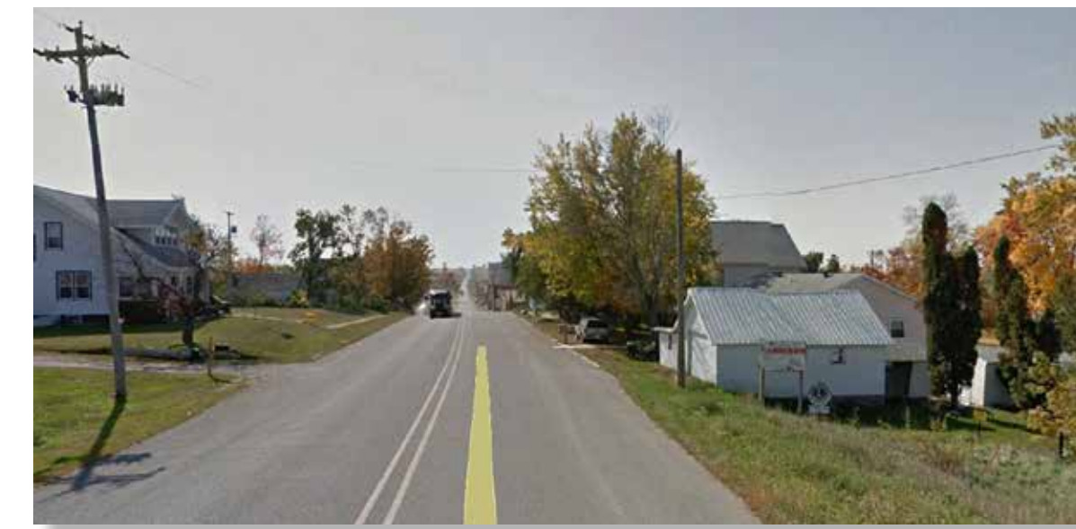
Sycamore Avenue existing conditions on north end of town.
