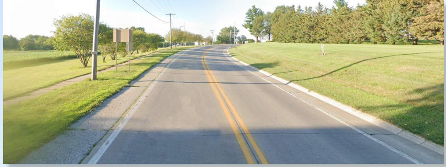
Existing view of Highway 151 looking south
