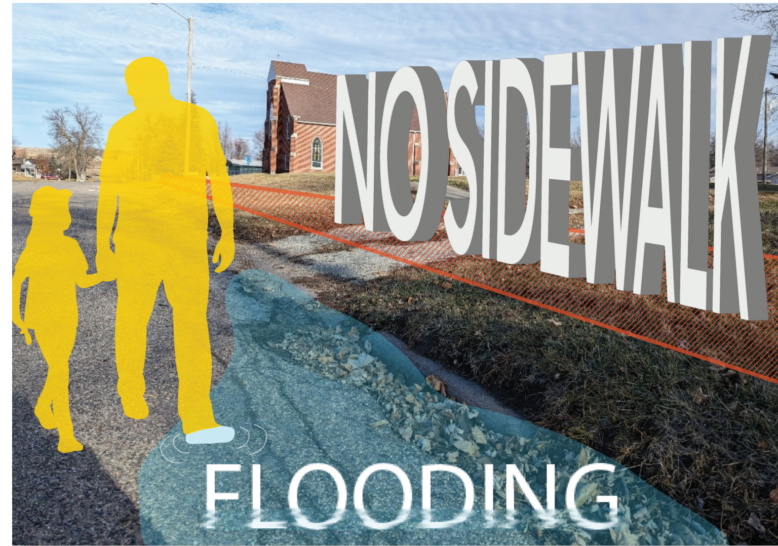
Potholes, the crowned roadway, flooding, and inferior sidewalks make Kilworth Street hard to navigate for all modes of travel.
