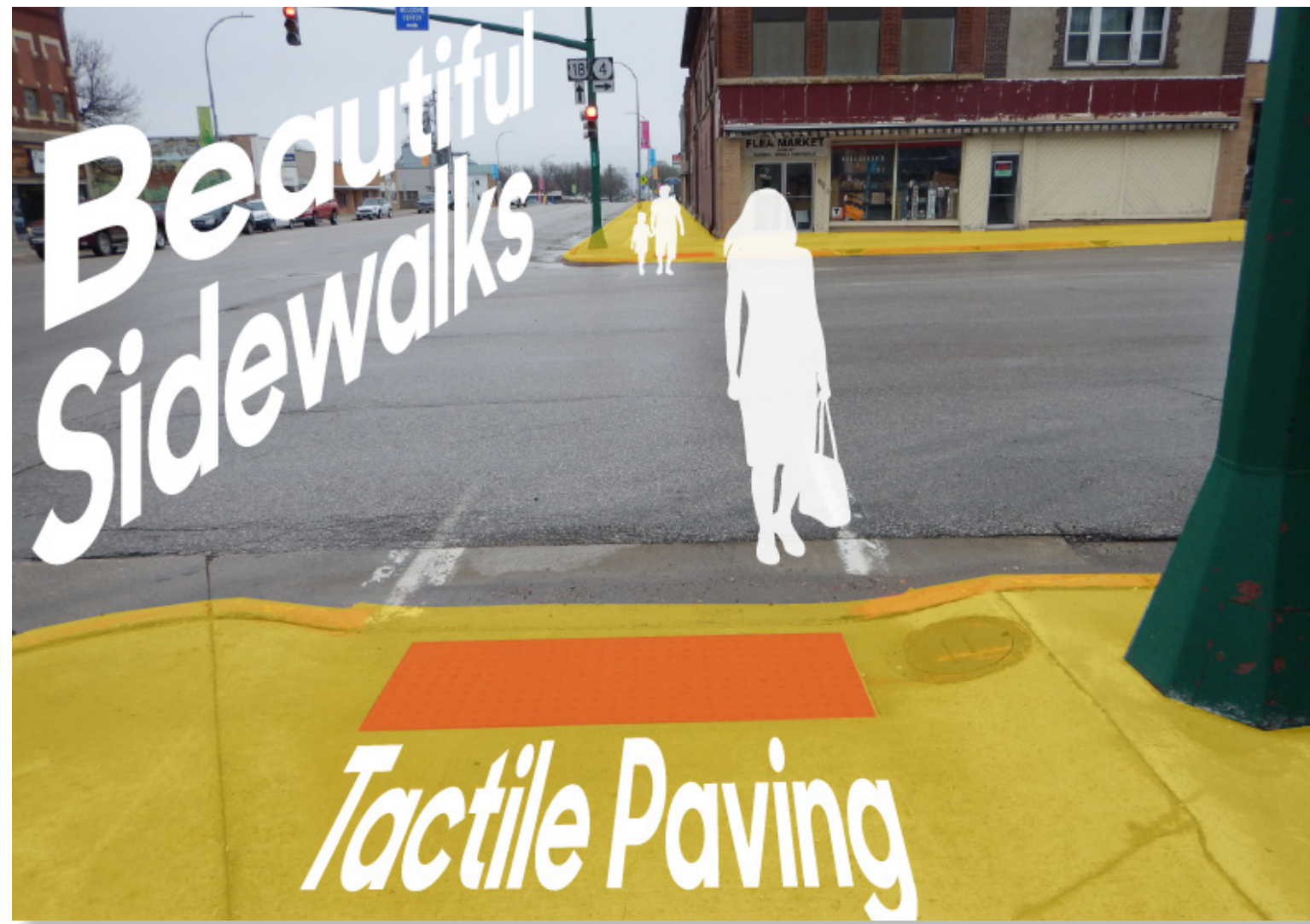
Residents appreciate the new sidewalks along Highways 18 and 4 because of the curb ramps and tactile paving.
