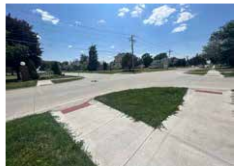
An example of a complete intersection with curb ramps and ADA tactile warning panels. Complete intersections are primarily on Connell and Clark Streets, which serve as primary routes for children to walk to schools.
