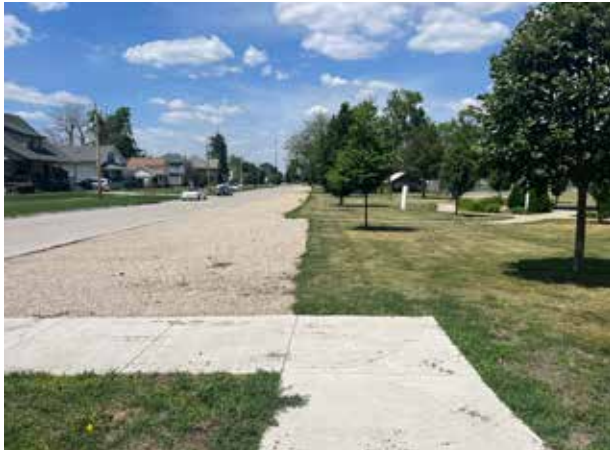
Existing conditions along Crismon Street
