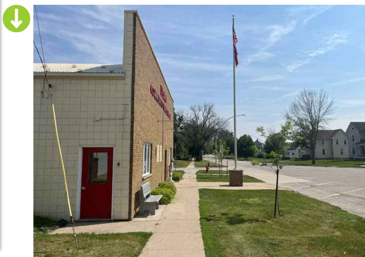
Existing sidewalk on Main Street looking south.
