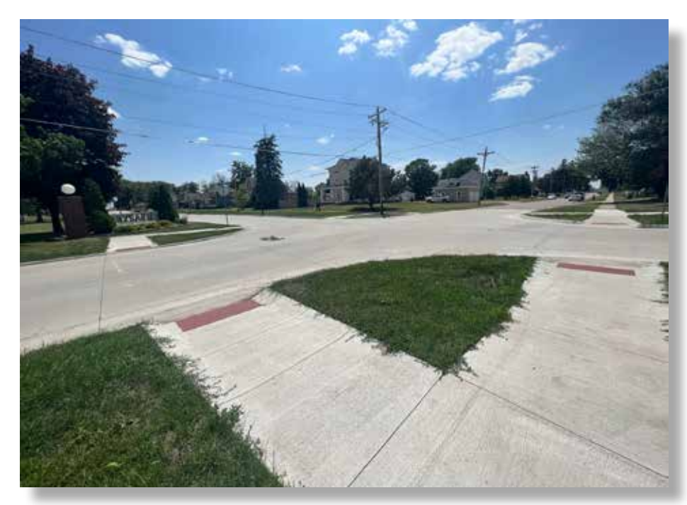
An example of a complete intersection with curb ramps and ADA tactile warning panels. Complete intersections are primarily on Connell and Clark Streets, which serve as primary routes for children to walk to schools.
