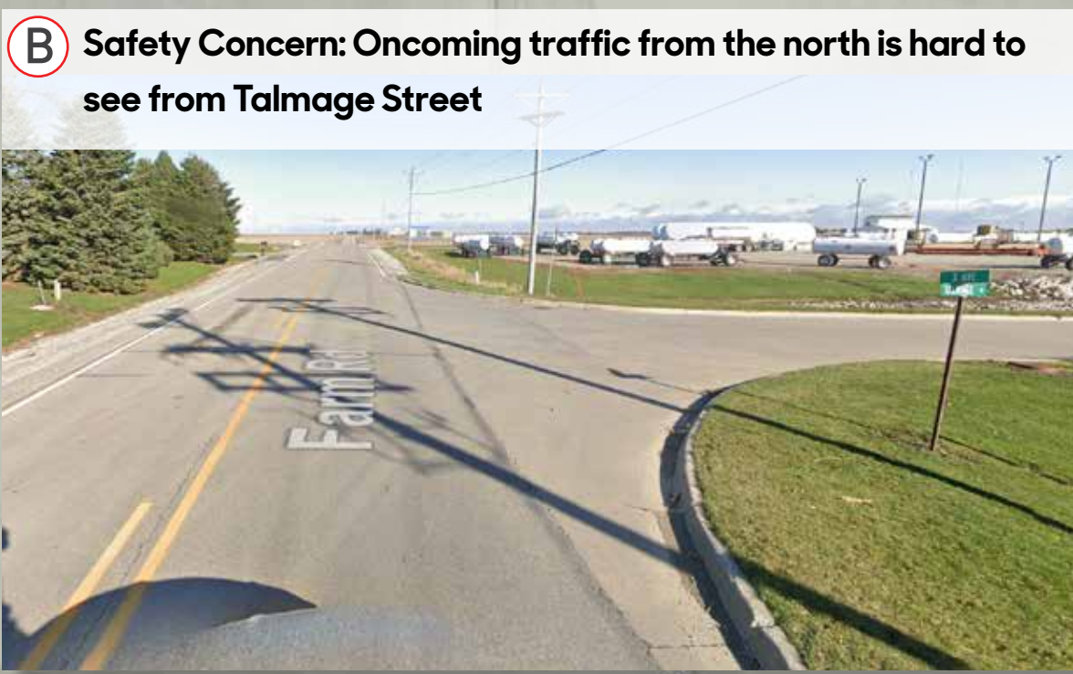
B Safety Concern: Oncoming traffic from the north is hard to see from Talmage Street Intersection of X Avenue and Talmage Street Photo Credit: Google Maps
