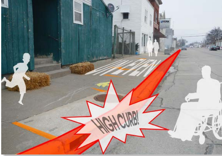
The sidewalks on Main Street are uneven and are difficult to access from the street because of the two-step curb, especially with snow in the winter.
