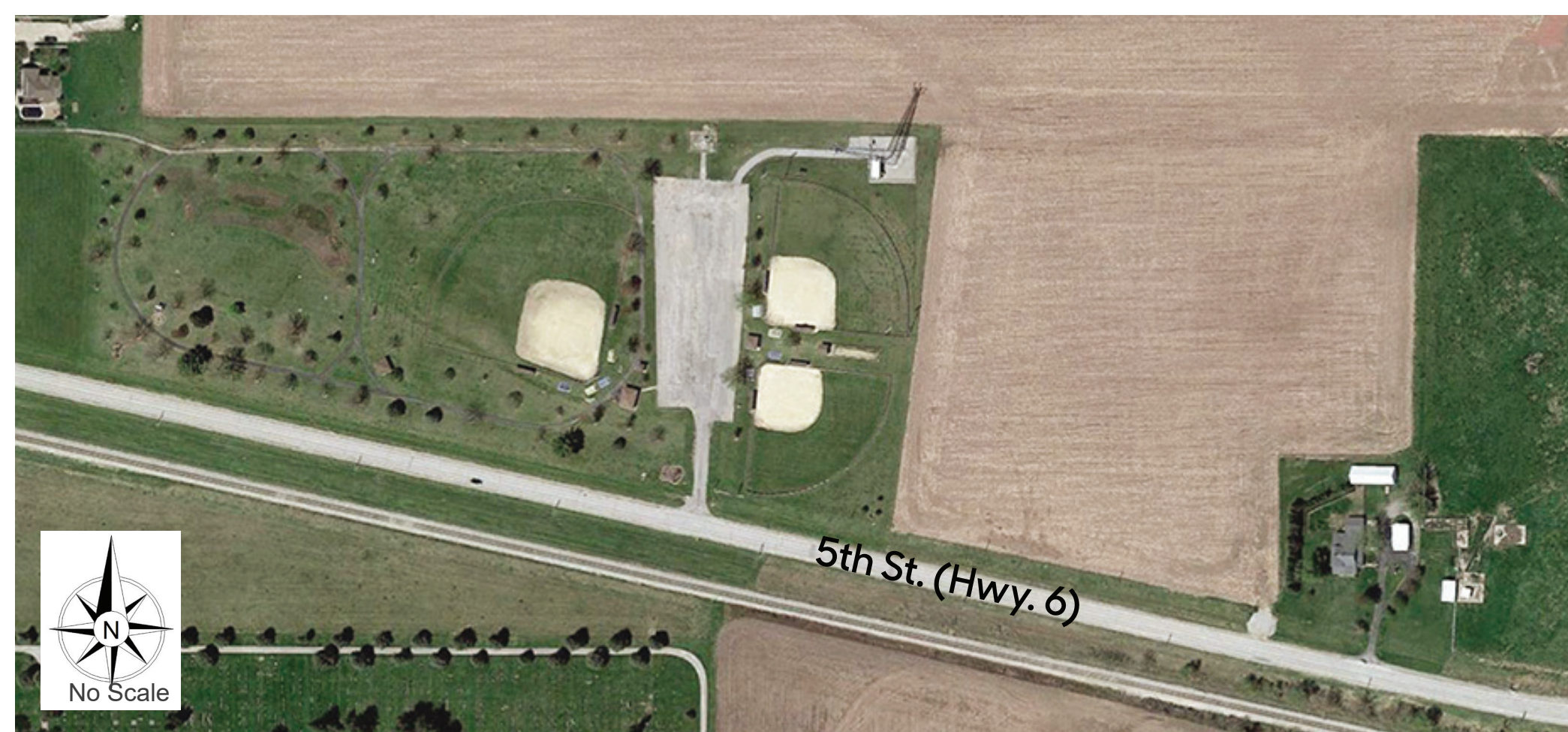
Existing aerial photo of Feldhan Park located along Hwy. 6 (5th St.) on the east edge of Durant
