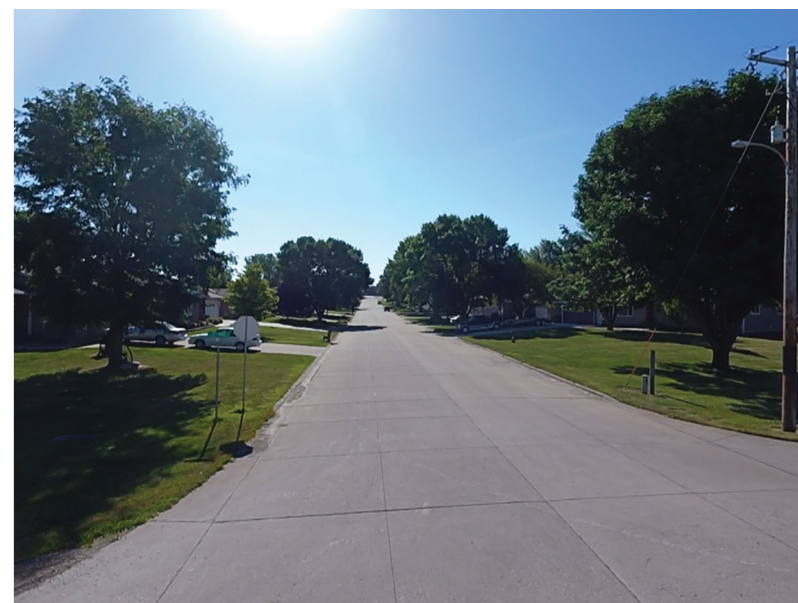
Existing 7th St. corridor looking east from 1st Ave.
