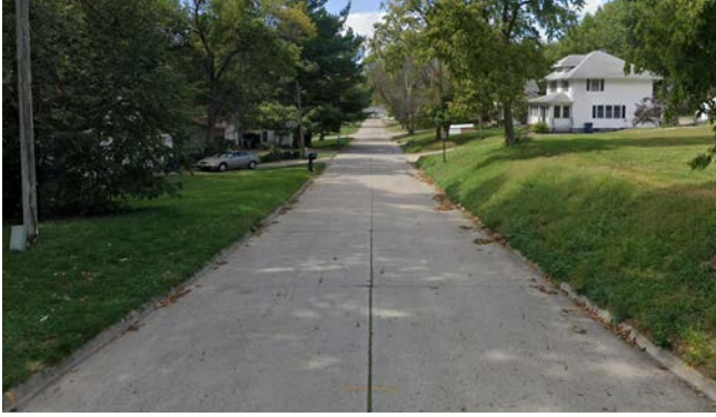
Existing - 3rd Ave S (Looking West)
