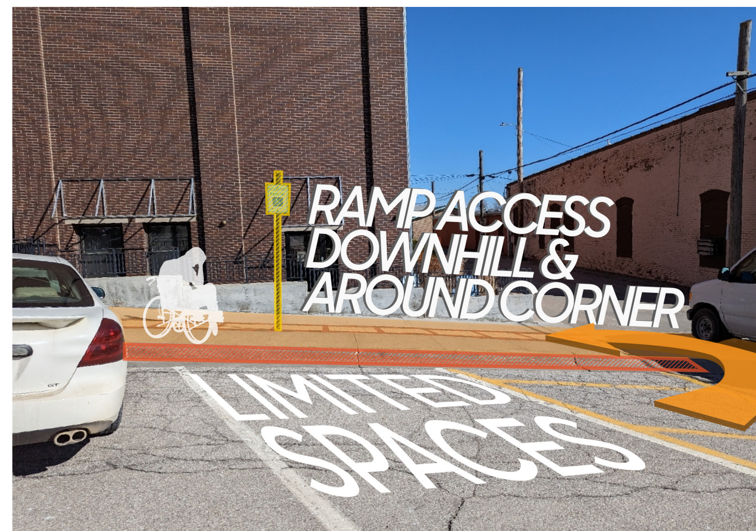
Uptown has only a few handicapped parking spaces that accommodate side-loading vans; some ramps are located around the corner, requiring the mobility challenged to travel on the street.
