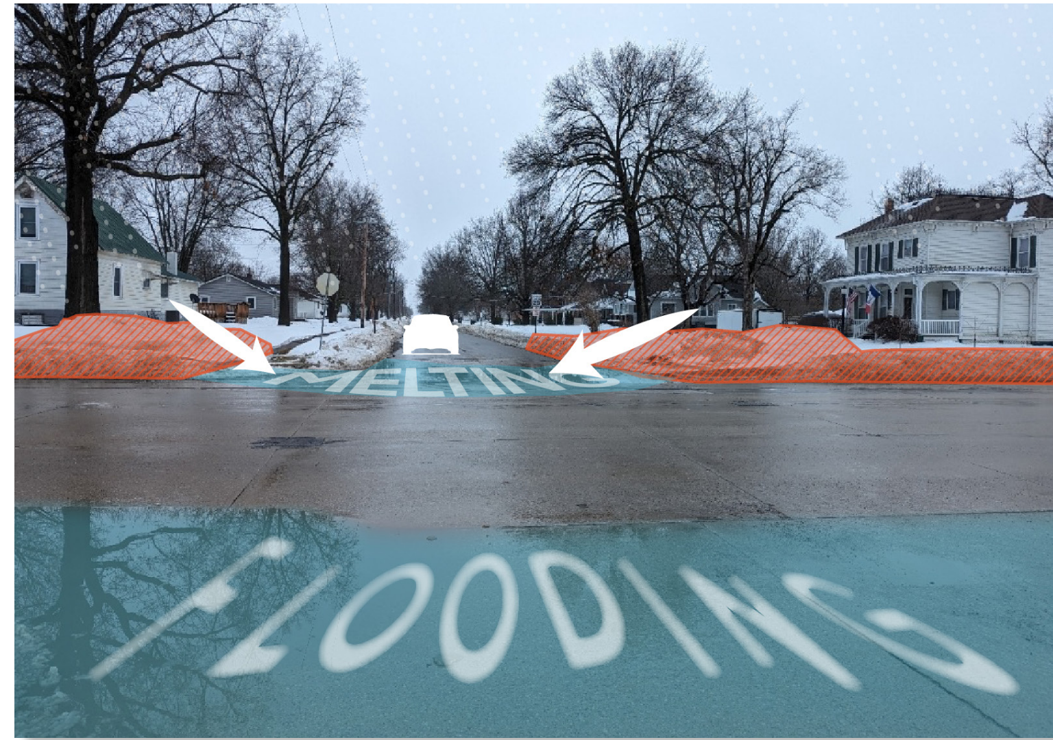
The intersection of Highway 2 and West Street floods after a heavy rain or snow melt because of a dip in the road and the absence of a storm drain.
