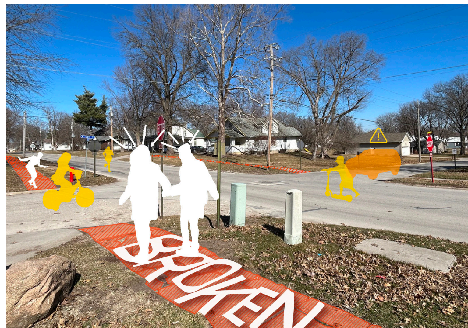
People walk in the roadway on South and West Streets because the sidewalks are either broken and uneven or missing altogether.
