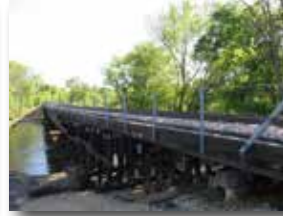
Historic Train Trestle Bridge
