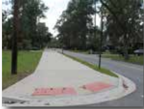
Ten-Foot Sidewalk With ADA Curb
