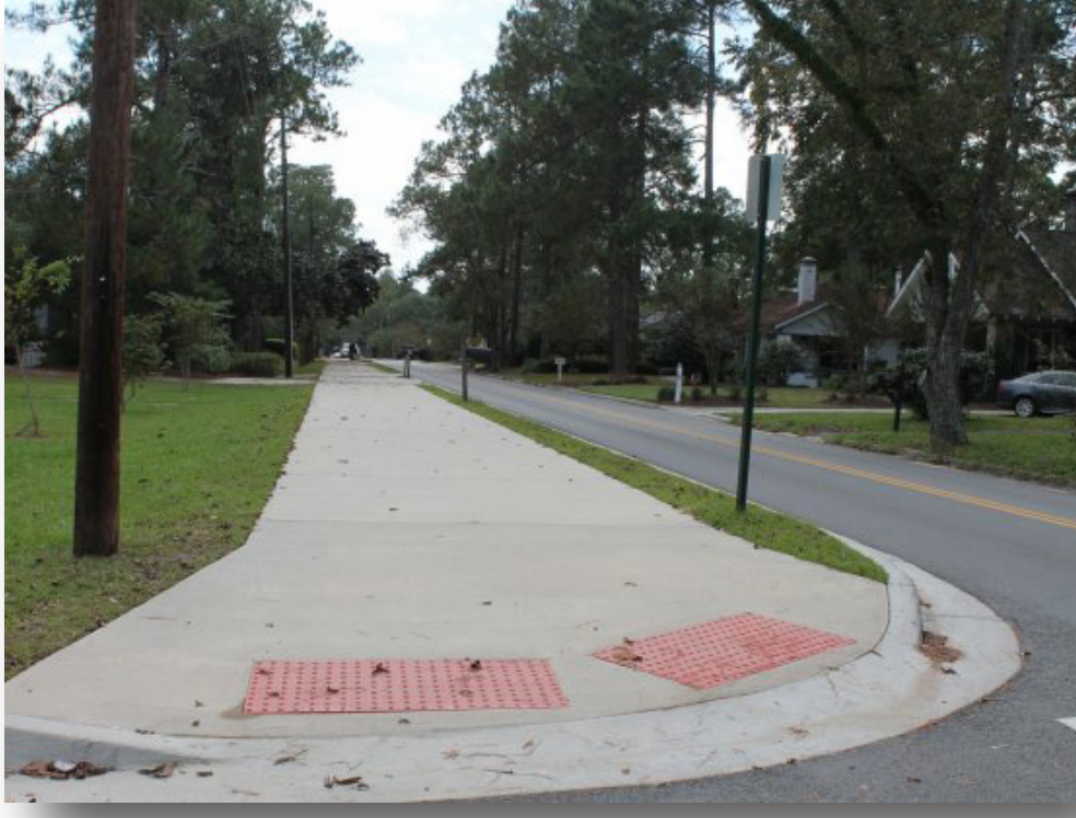
Ten-Foot Sidewalk With ADA Curb
