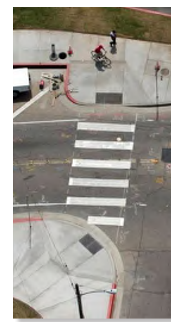
Pavement markings at crosswalks
