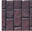
Example 12f: Decorative pavement (laid & stamped concrete).
