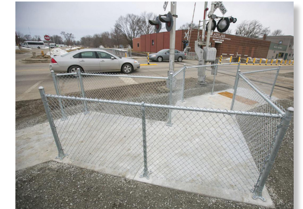
Example 16f: Restricted channelized pedestrian crossing
