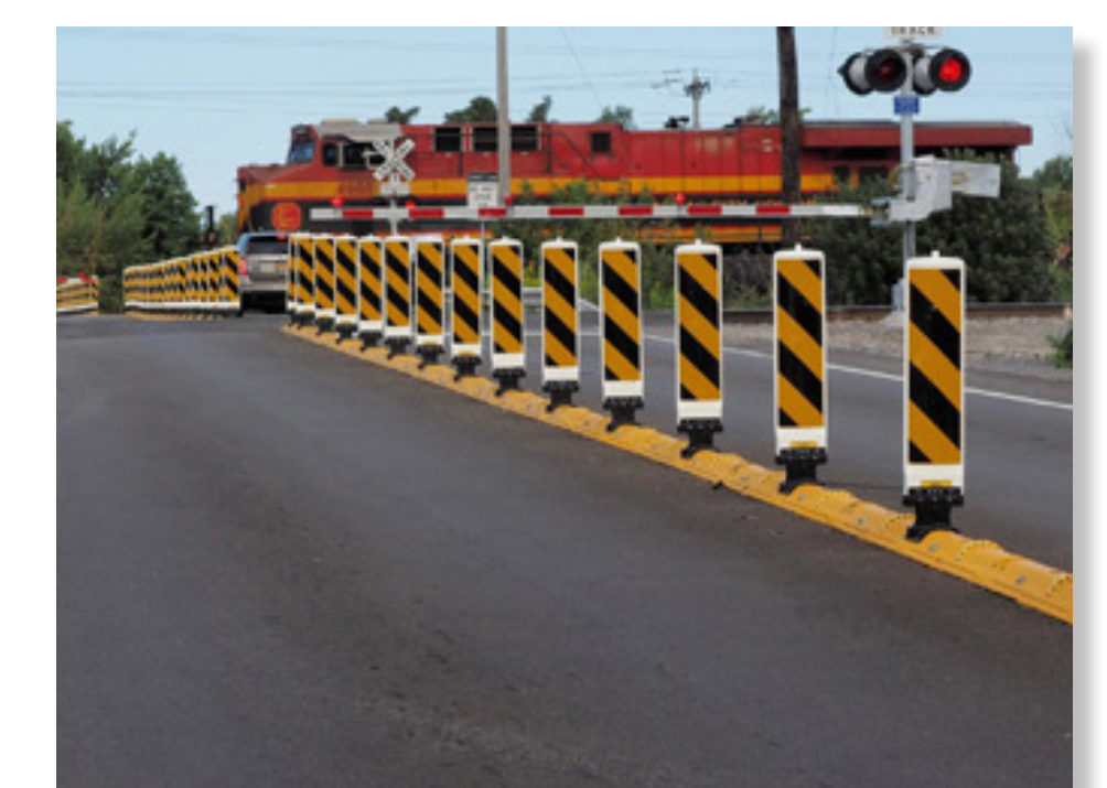
Example 16e: Gates with channelization devices
