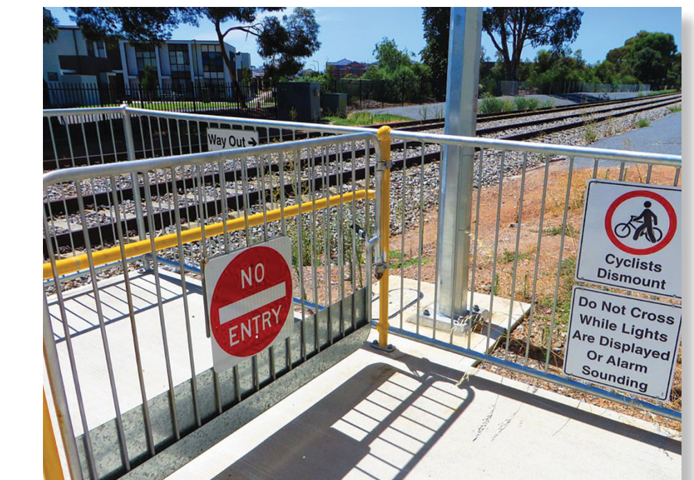
Example 16j: Automatic gate control for pedestrian crossing
