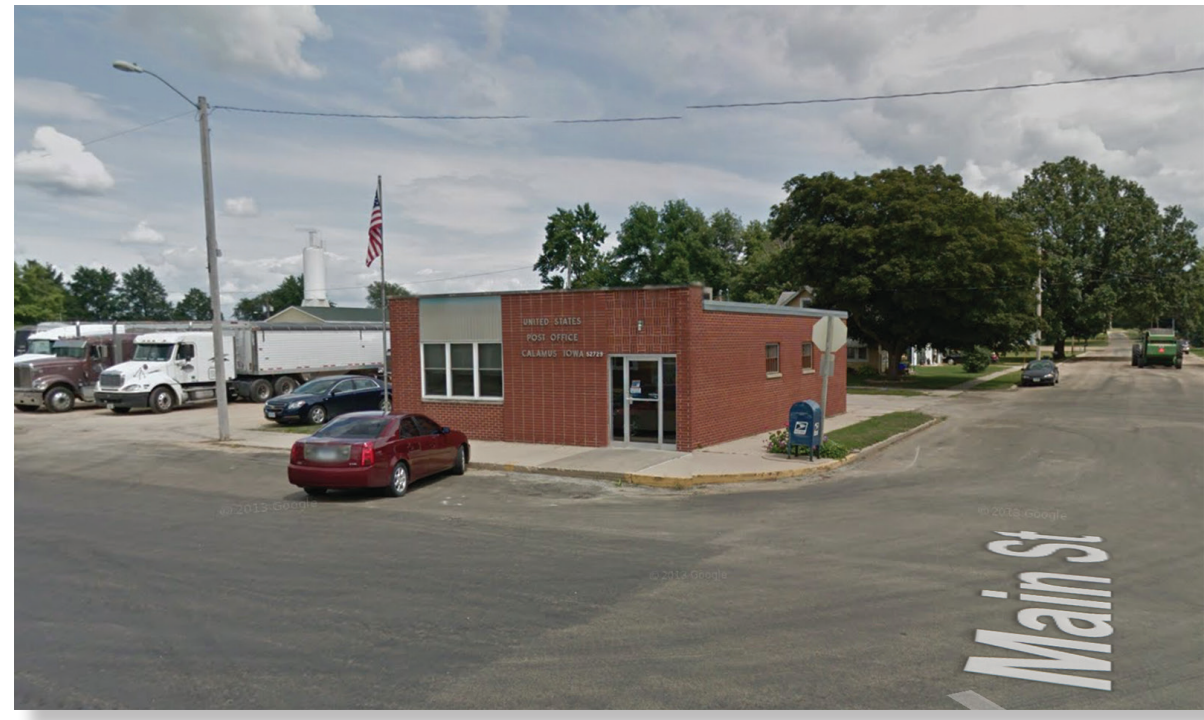
Existing photo 13a: Photo taken from 2nd St. & Main St. intersection looking northeasterly towards the post office
