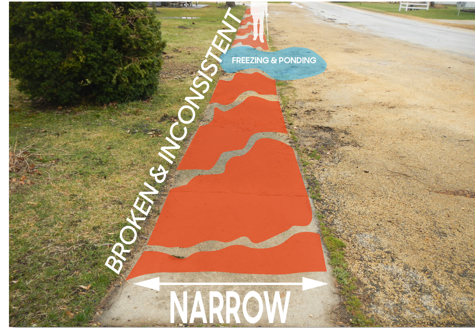
The sidewalks along 2nd Street are narrow, broken, and inconsistent causing residents to walk in the street.
