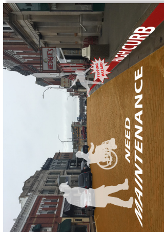
The high curbs on Main Street cause accessibility issues for multiple user groups.
