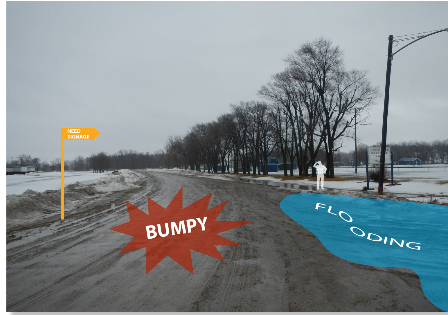
The roads around the baseball field are in poor condition, and often flood.
