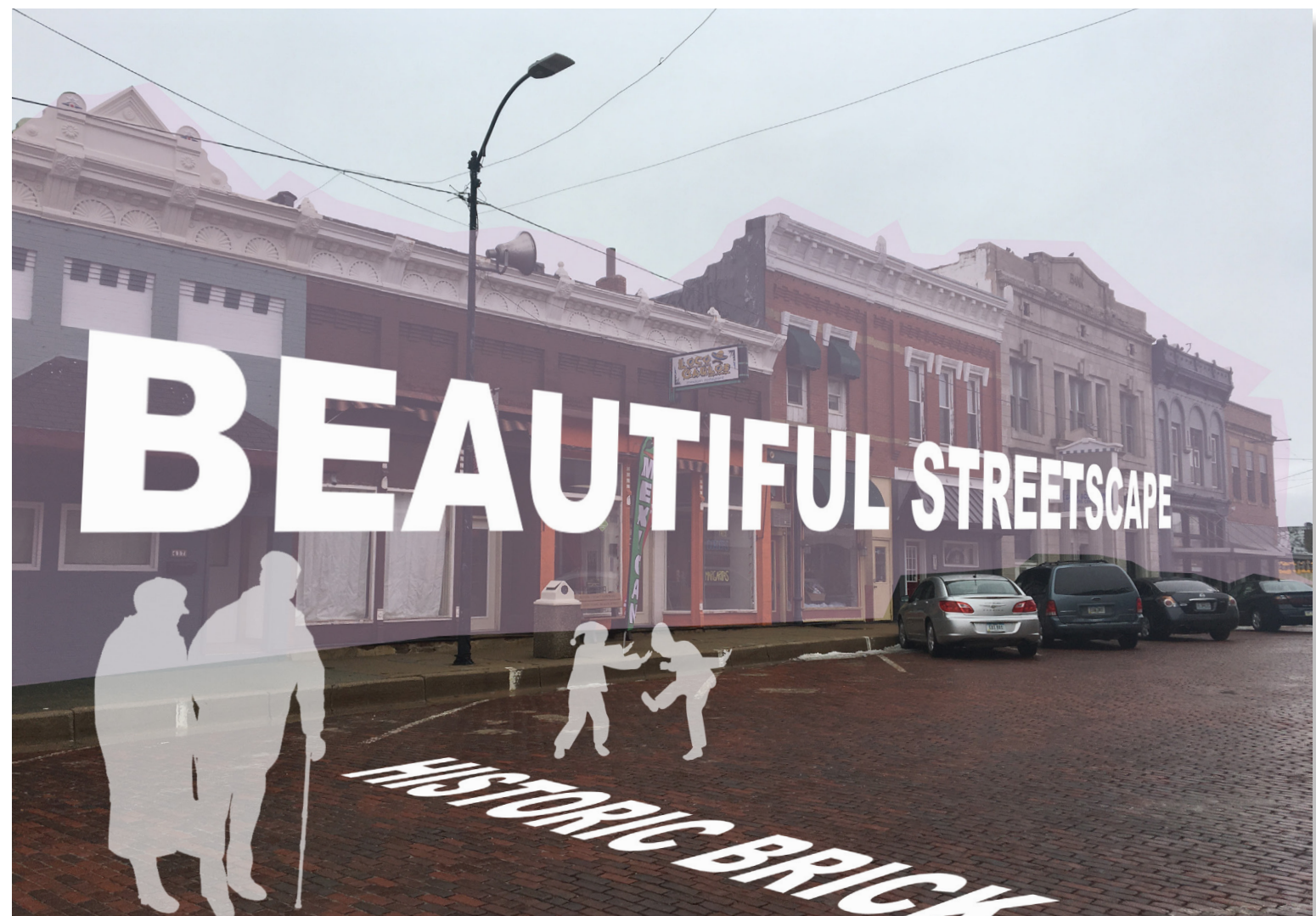
The brick streets in town have historic value and make for beautiful streetscapes as long as they are well maintained.
