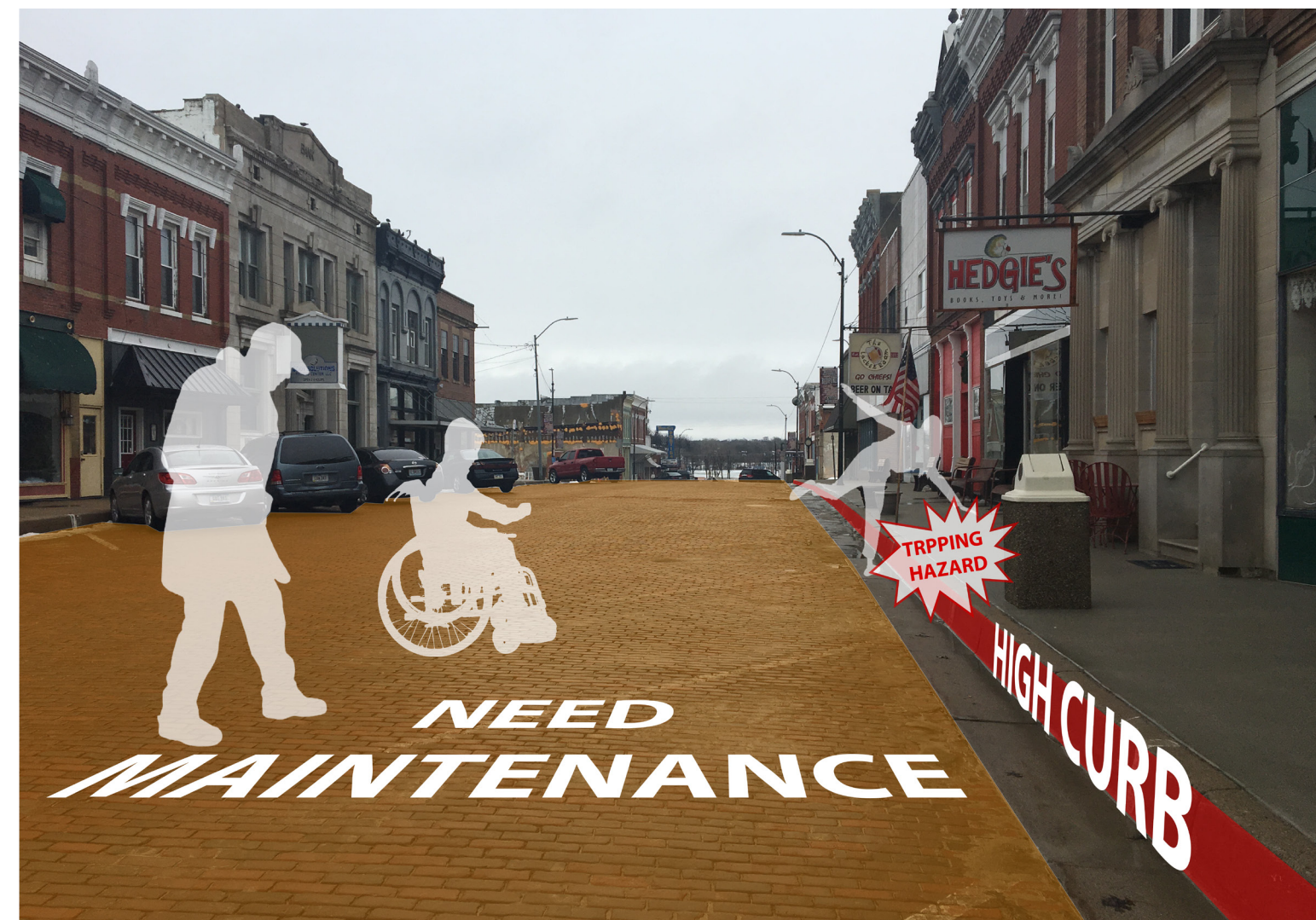
The high curbs on Main Street cause accessibility issues for multiple user groups.
