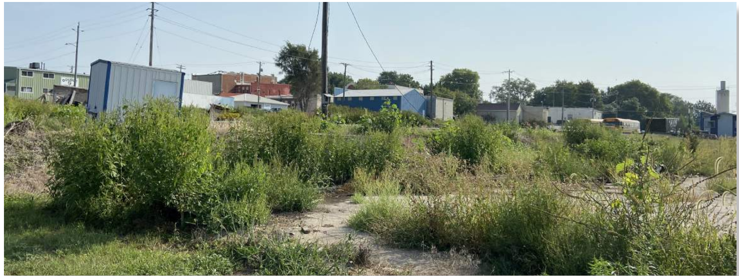
Existing view of silo foundations looking northeast
