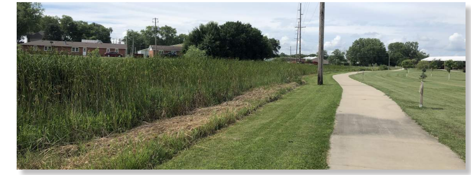
Existing view looking south from trail at stormwater swale
