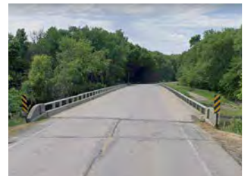
6 Crossing East Fork Des Moines River
