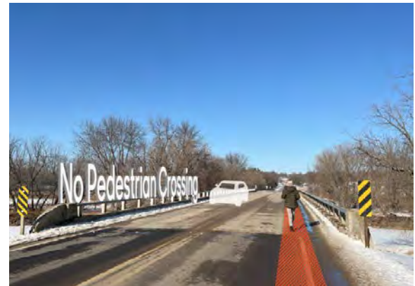
Lack of sidewalks at the bridge over the river on Orton Road creates a disconnect between town and the neighborhood and park to the southwest.
