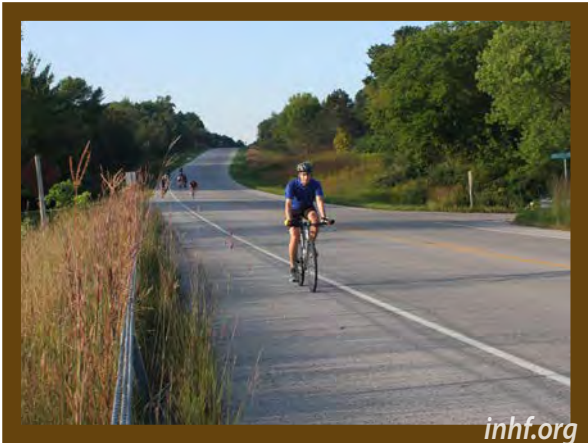
Increasing road-shoulder width, whether paved or granular surface, is an important component for bike safety. These paths are typically used for recreation or destination activities, and many events such as RAGBRAI follow highways and rural roads.
