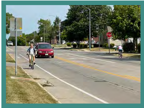
Bike lanes are dedicated routes within the street for cyclists. They utilize markings and/or painted surfaces to bring attention and importance to the cyclist area. They can also be protected from traffic through barriers and buffers between the bike lane and adjacent traffic.
