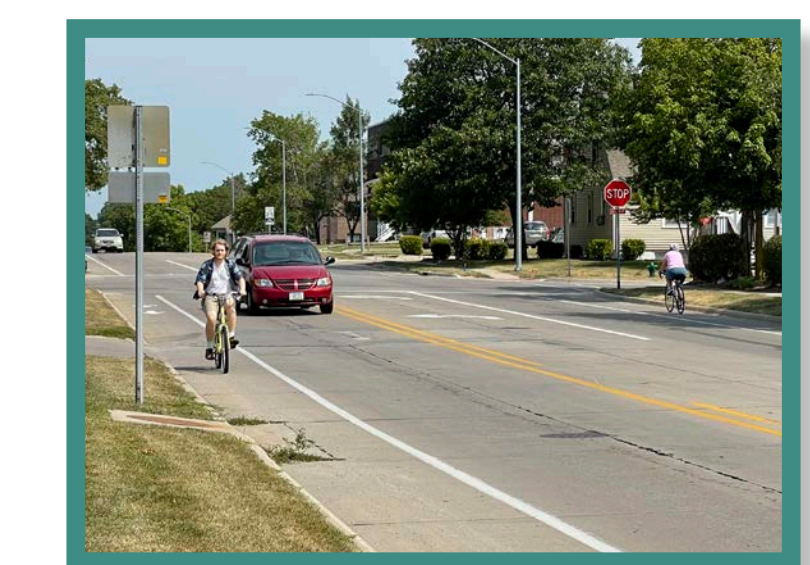
Bike lanes are dedicated routes within the street for cyclists. They utilize markings and/or painted surfaces to bring attention and importance to the cyclist area. They can also be protected from traffic through barriers and buffers between the bike lane and adjacent traffic.
