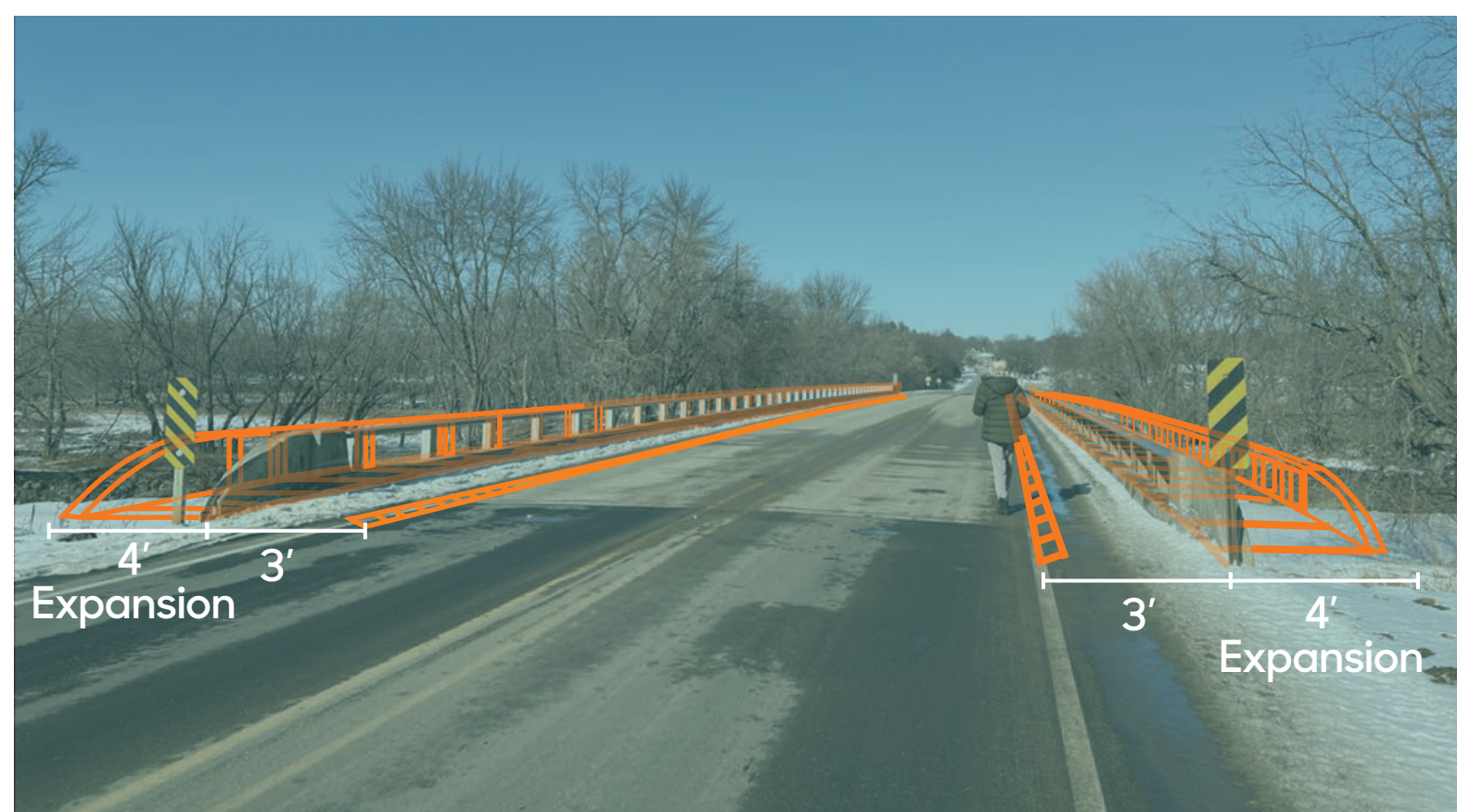
Potential Orton Road bridge expansion would accommodate a 6' wide bike lane on each side with a painted buffer
