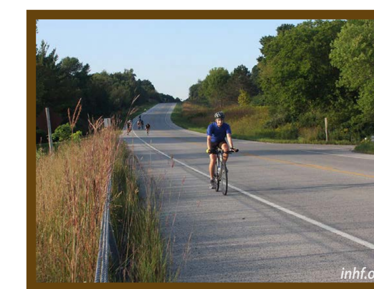
Increasing road-shoulder width , whether paved or granular surface, is an important component for bike safety. These paths are typically used for recreation or destination activities, and many events such as RAGBRAI follow highways and rural roads.
