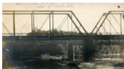
G - RRVT- Adel Bridge
