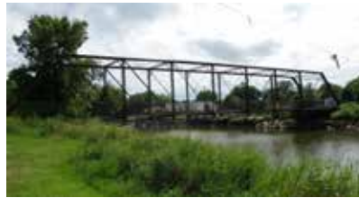
E - Wiscotta Bridge
