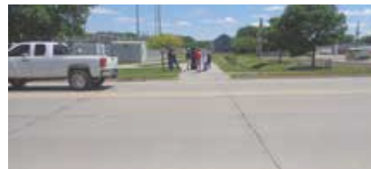
Existing unmarked trail crossing at HWY 169
