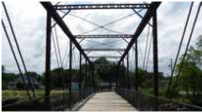
E - Wiscotta Bridge
