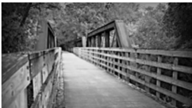
G - RRVT- Adel Bridge
