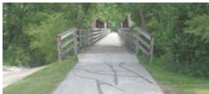
RRVT Bridge at The Raccoon River
