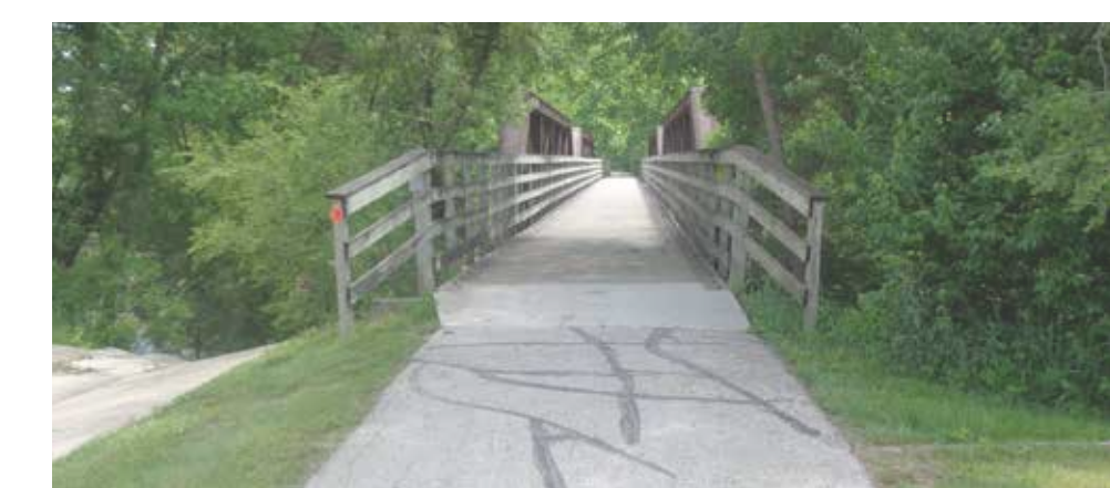
RRVT Bridge at The Raccoon River
