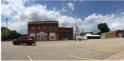
The west side of Main Street currently has multiple open lots with more to follow, as the old bank building is taken down. The remaining parcels will provide an open green space that could have a temporary life as a park like space. Future vision for this site would include the development of businesses, but open space could remain in key locations. The steering committee's goal for this site was to develop a landscape treatment that could be temporary or permanent to allow future structures to be built.
